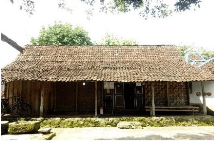
Fig. 10. A simple commoner's house in Java. One building on a low compacted soil platform, and a simple kampung style roof. [Source: Muqoffa]
