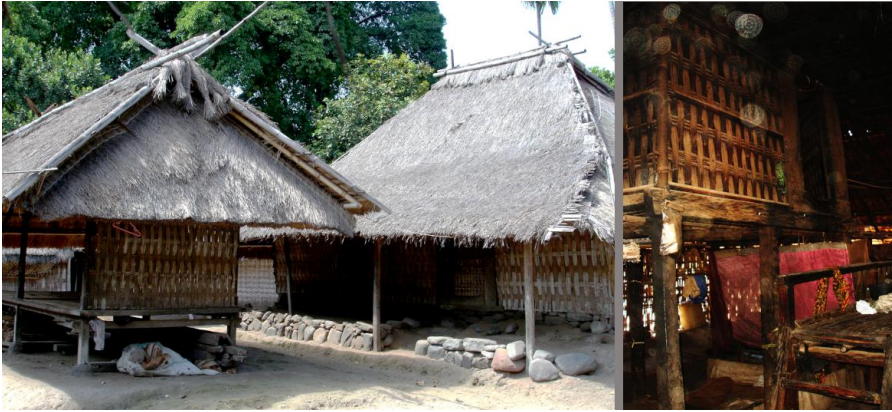
Fig. 6. The berugaq and the bale in Segenter Village, from Lombok. Inside the bale is the inan bale (mother of the house) a closed raised floor at the center, used as a sleeping place for virgins of the house, and family heirlooms. [Source: Author]
