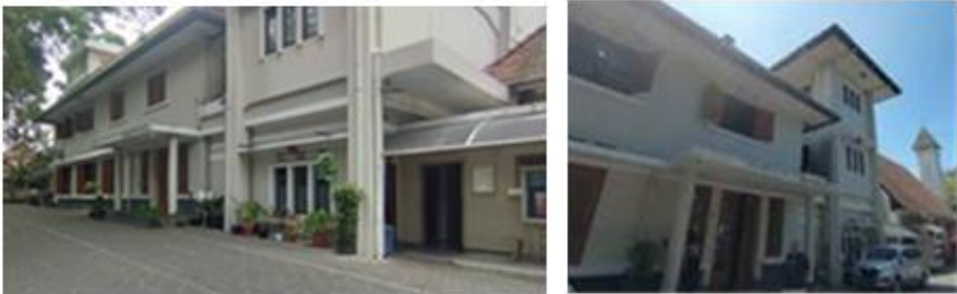
Fig. 10. The Rectory building at the back side use the same colour as the Church
