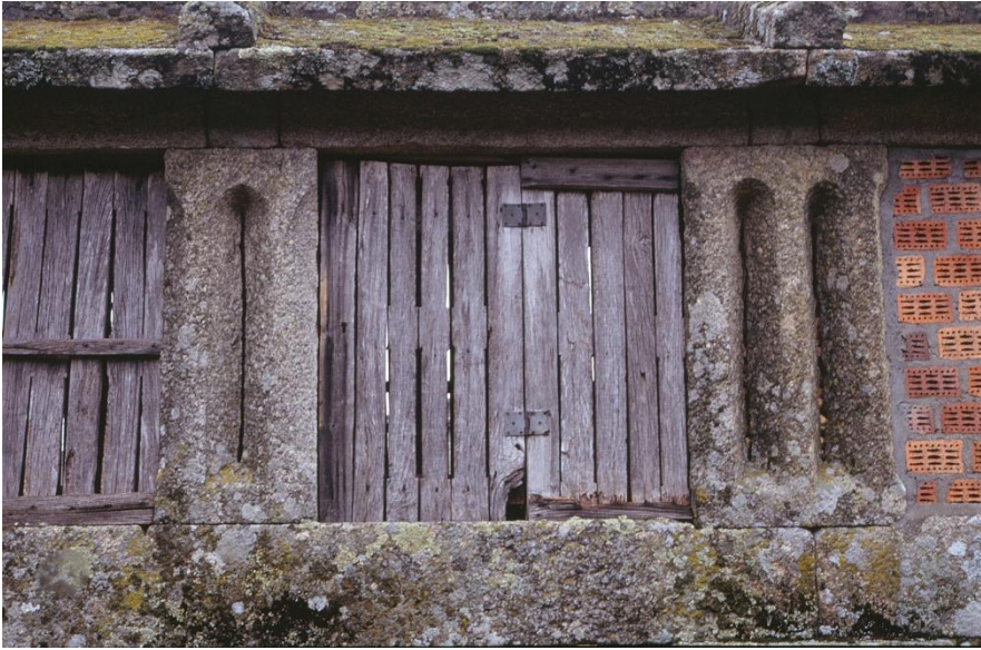
Fig. 8. Detail of the wall of a granary from Lindoso showing two supporting stone studs with slits. The one with two slits is most similar to a triglyph as seen in Figure 6. Photo G. Domenig, 1989
