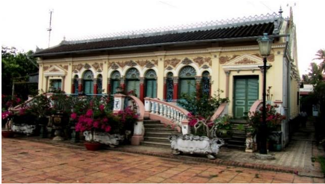
Fig. 10. Binh Thuy Ancient House is located at No. 142-144 Bui Huu Nghia Street, Binh Thuy Ward, Binh Thuy District, Can Tho City. First built by Duong Van Vi with a wooden house, tiled roof in 1870. After 30 years of use, the house was completely designed and built in 1911, the exterior has a classic French style but the interior still retains the ancient architecture. (Source: Author, 2011).
