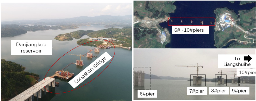
Fig. 1. The substructure construction of Longshan Bridge
