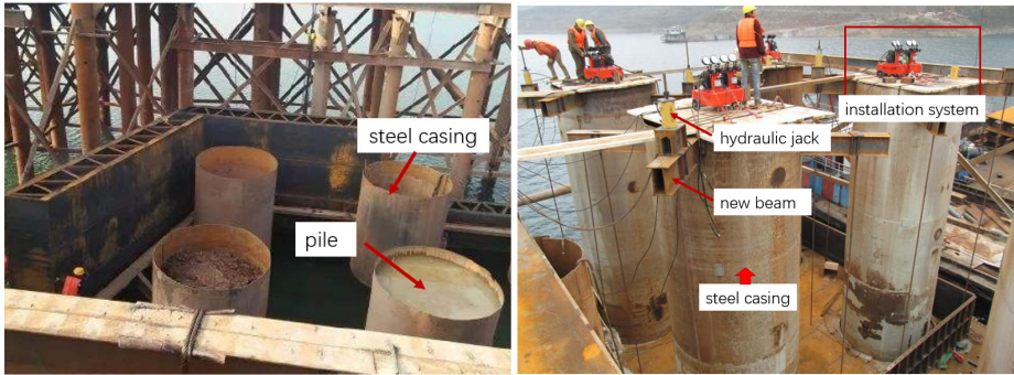
Fig. 2. Location of the boxed cofferdam
