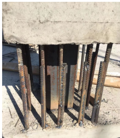
Fig. 14. Welding Effect of Vertical Reinforcements
