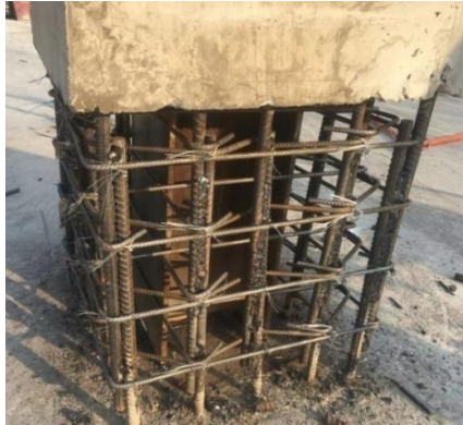
Fig. 15. Binding of Stirrups at Prefabricated Column Bottom
