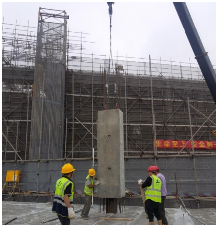
Fig. 12. Prefabricated Column Hoisted in Place
