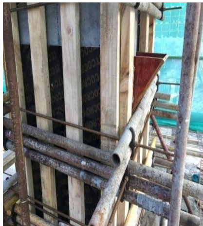
Fig. 16. Mold and Bellmouth Installation for Joint
