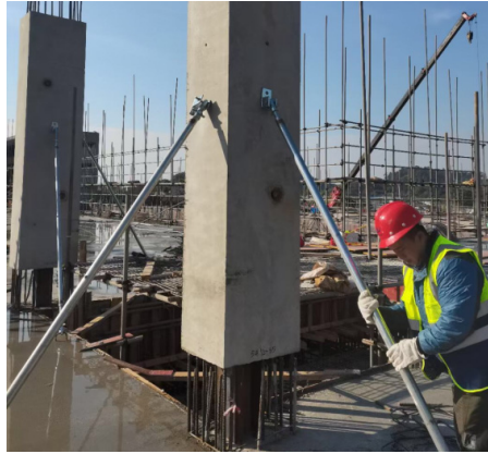
Fig. 13. Setting up of Diagonal Bracing on Prefabricated Columns
