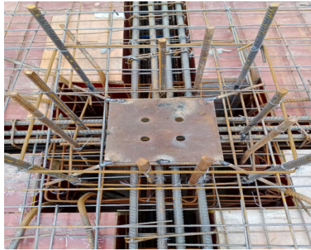
Fig. 11. Welding of Embedded Steel Plates at Column Bottom
