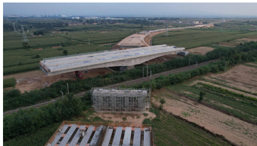
Fig. 1. Rotational bridge construction site diagram.
