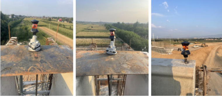
Fig. 12. Installation Diagram of the 360° Prism at the Cantilever End of the Main Girder
