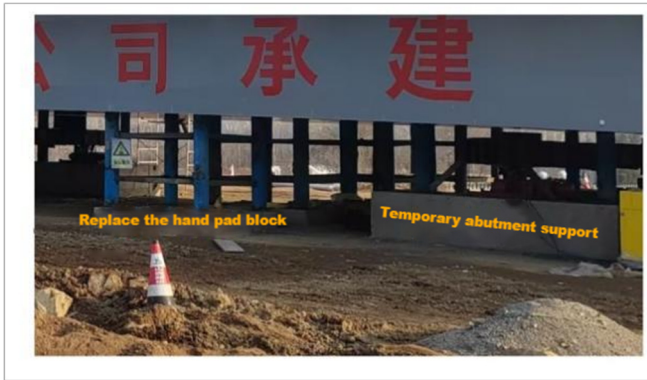
Fig. 4. Temporary support on-site layout diagram.
