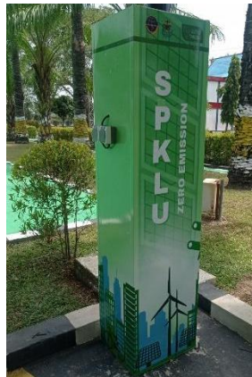
Figure 4 Construction of the cover and battery compartment
