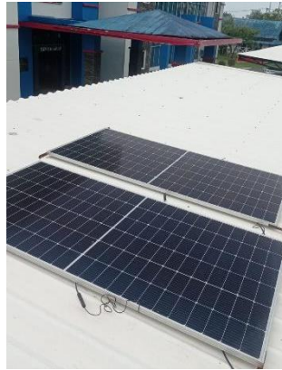
Figure 5 Installation of solar panels and testing
