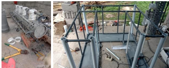
Figure 4. Construction of Filtering Equipment
