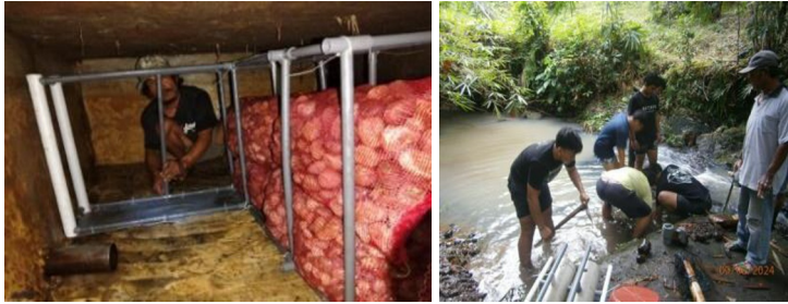
Figure 5. Installation of Filters
