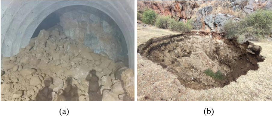
Fig. 2. Karst cave at DL I 68+347 of Qinhe Tunnel.
