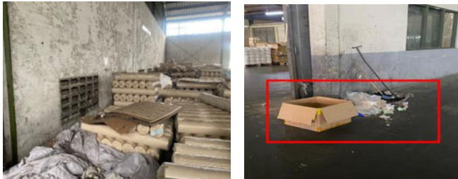
Fig. 1. Warehouse section condition.
