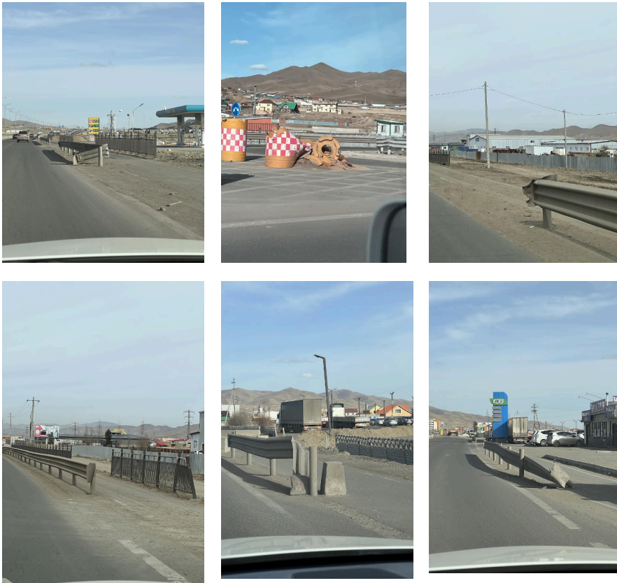
Fig. 1. The current condition of safety railings (guiderail) conditions.
