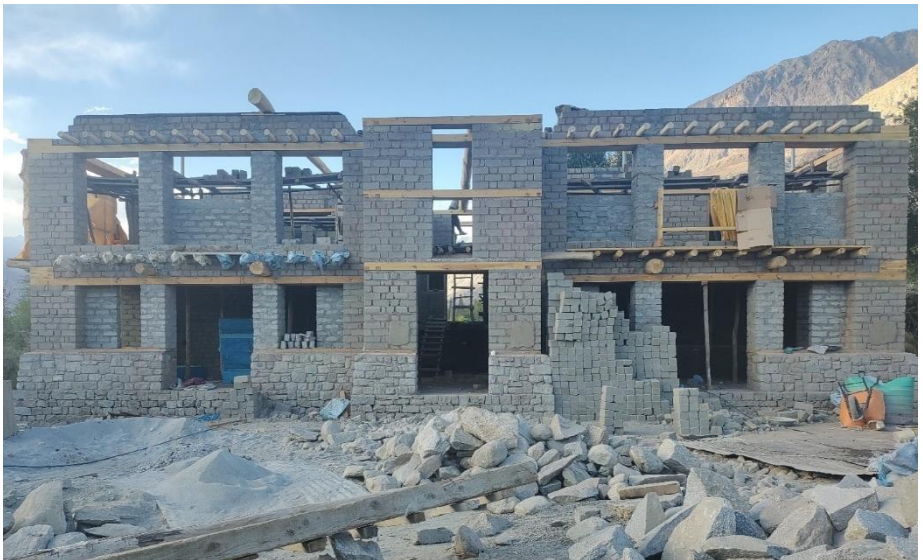
Fig. 12. Modern day usage of taq techniques in North India
