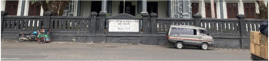
Fig. 4. Massive Perimeters Infront of the Building
