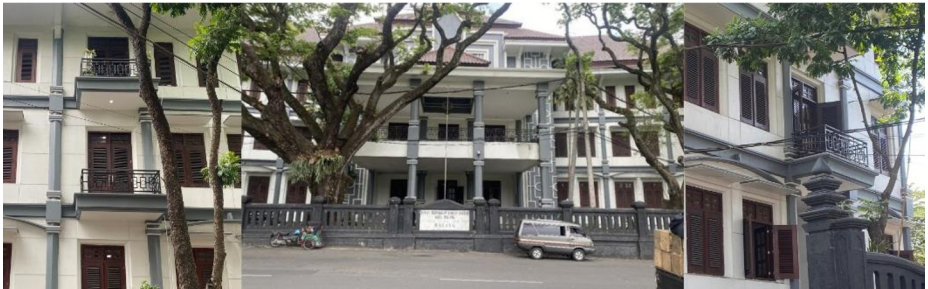
Fig. 9. Building Front and Side Balcony
