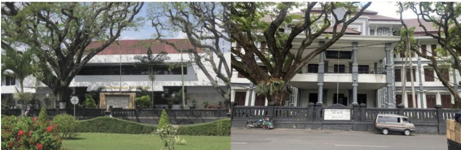
Fig. 3. Building Facade Before & After 2012
