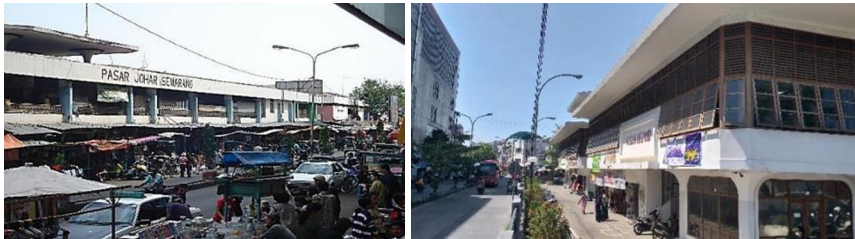
Fig. 5. (Left) Pasar Johar in 2007; (Right) Pasar Johar in 2022 (source: Kiswari et al., 2022)
