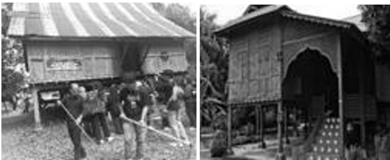
Fig. 6. The typology of buildings with sloped roofs in Malaysian local architecture underscores the importance of roof space and layered roof structures, with the roof form often extending upward in a pronounced vertical expression. The use of natural materials such as straw, bamboo, clay tiles, and wooden shingles creates cross-ventilation gaps at the intersections between the upper and lower roof layers. This typological pattern is further reflected in the presence of both grounded (landed) and raised (stilted) building forms. (Source: Author).
