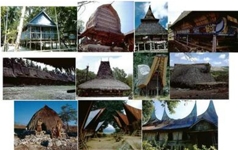
Fig. 4. The typology of buildings with sloped roofs in Indonesian local architecture highlights the importance of roof space and layered roof structures. These roofs often rise upward in a distinctive vertical expression. The use of natural materials such as straw, bamboo, clay tiles, and wooden shingles creates cross-ventilation gaps at the junctions between the upper and lower roof levels. In addition, both grounded (landed) and stilted (raised) building forms are commonly found (Source: Roxana).
