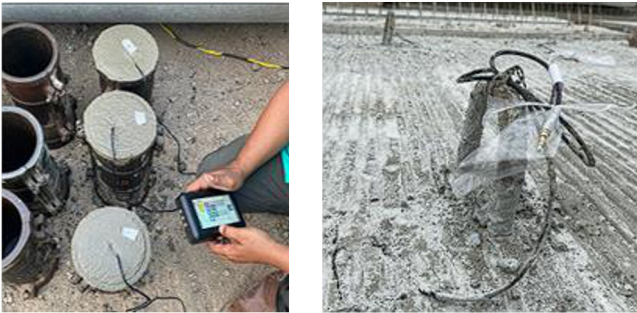
Fig. 6: Concrete Maturity Test Portable Type Instalment and the sensor attached
