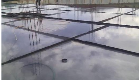
Fig. 2. Image depicting enormous water requirement associated with conventional concrete curing
