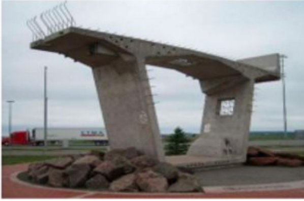
Fig. 1. Display of a typical segment of the Confederation Bridge [9] ( https://doi.org/10.3390/s21134336 )
