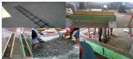
Fig.3. Casting RC beams
