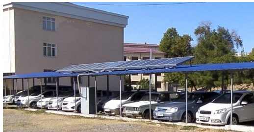
Fig. 1. General view of the car parking area with nighttime lighting powered by a 2.7 kW PVPS
