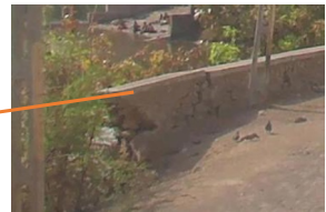
Walls around Lake
