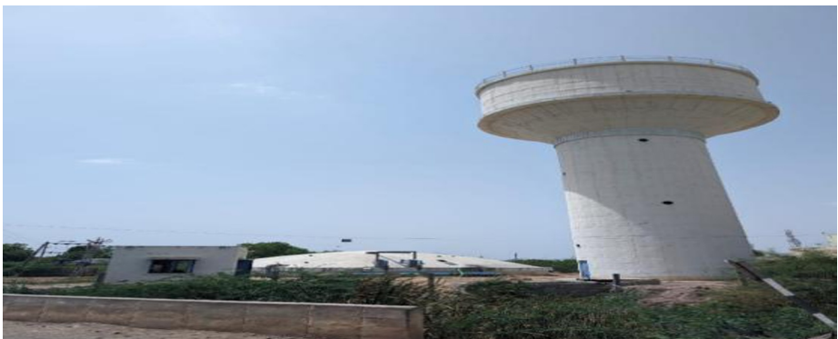
Fig.19. Image of existing overhead water tank
