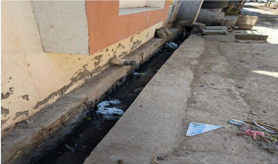
Fig.21. Existing Open drainage in village
