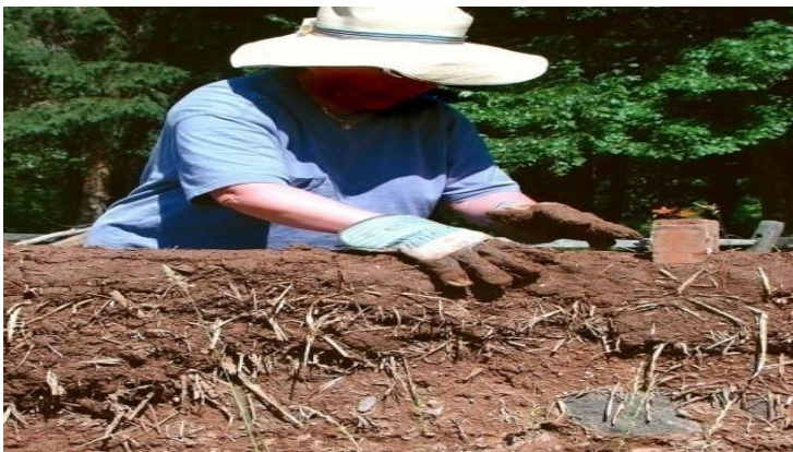
Figure 2(a): The mud and straw mixture for making homes in 1500 B.C
