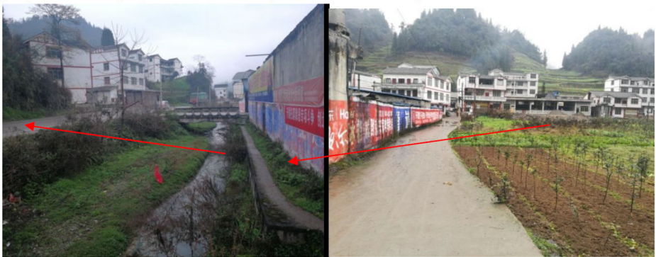
Fig. 3. Shallow-buried section of the tunnel underpassing buildings
