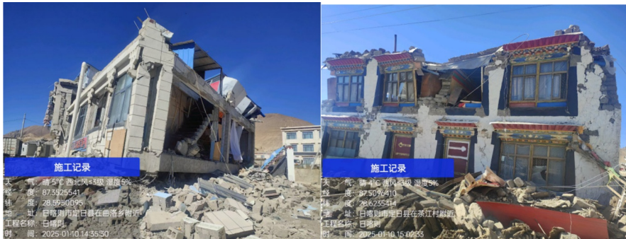
Fig. 4. Self-built housing Pictures
