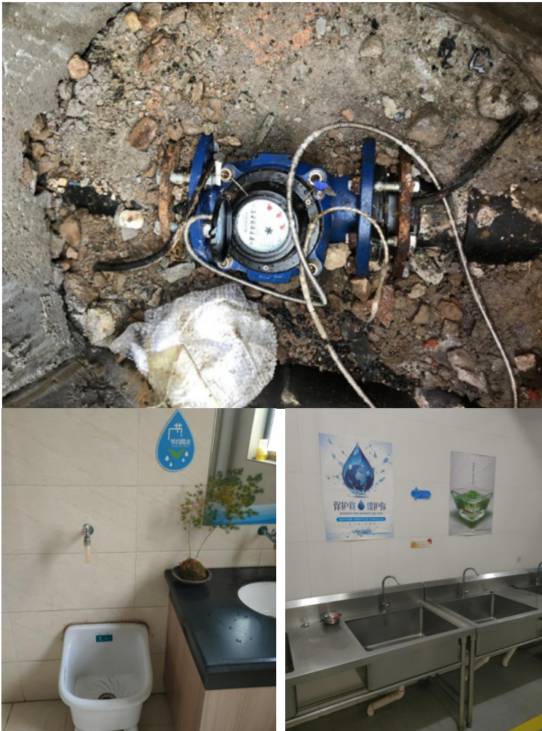
Fig. 4. Installation of metering facilities and water-saving appliances
