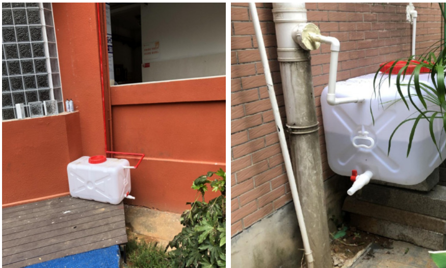
Fig. 5. Installation of unconventional water utilization facilities
