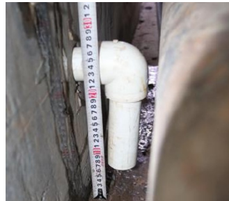
Fig. 6. Leak hole layout under downward leakage conditions.
