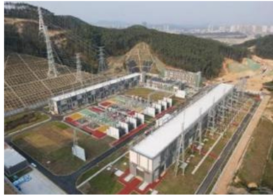
Fig. 1. The first "Near Zero Energy" dual carbon demonstration substation in China - Guangzhou 500kV Kebei Substation.
