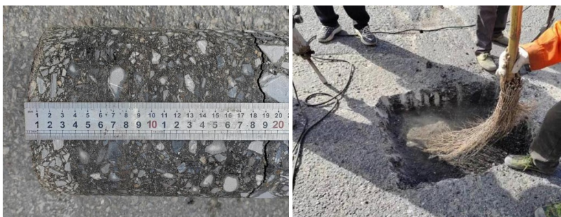
Fig. 2. Surface core drilling sampling and pit exploration test.
