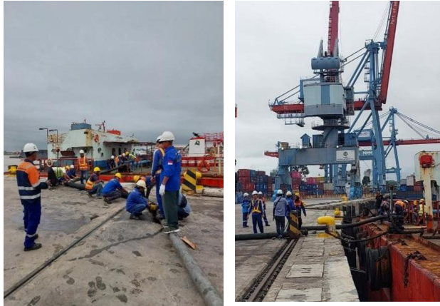
Figure 2. Implementation of Loading CPO onto Ships at Boom Baru Port, Palembang
