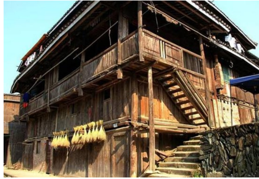
Fig. 1. Traditional Diaojiaolou (Stilted Building) in Chengyang Bazhai
