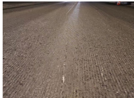
(b) Milled pavement surface
