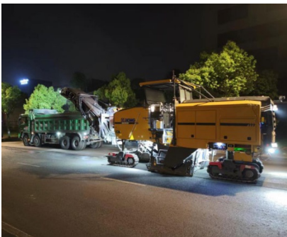
(a) During milling construction
