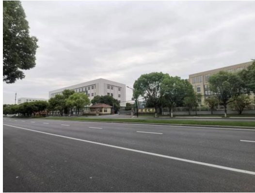
Fig. 10. Condition of Gaofuer Road after paving
