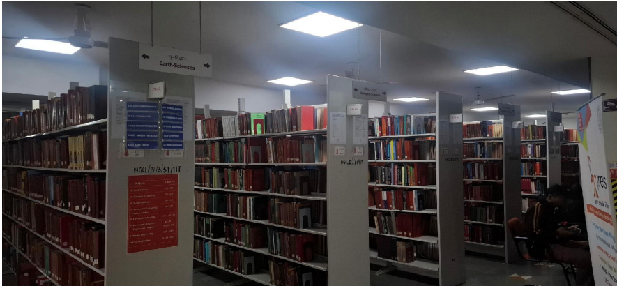
Fig. 12. Glare from Overhead Lighting
