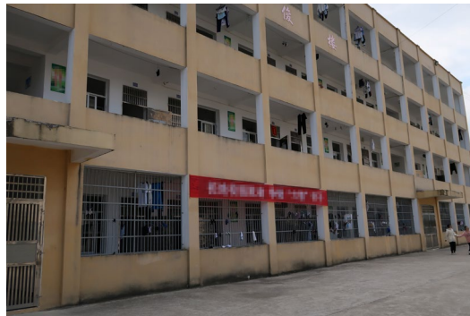
Fig. 1. Dormitory building of H School.
