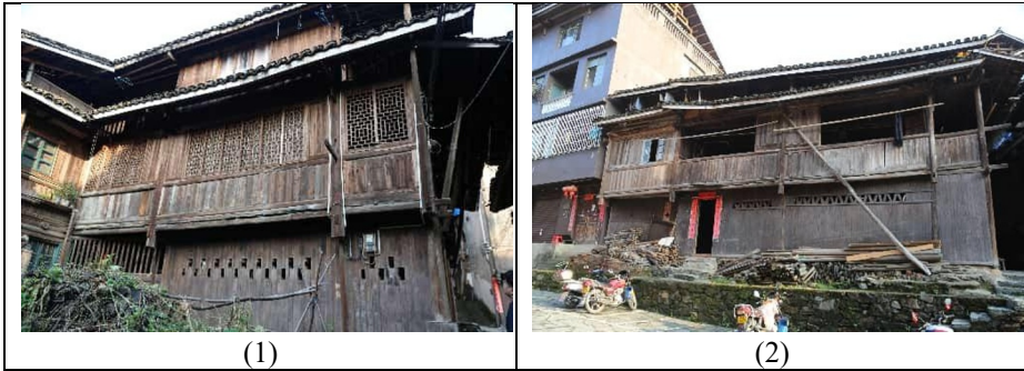
Fig. 1. Ganlan-style traditional architecture in Chengyang Eight Villages
