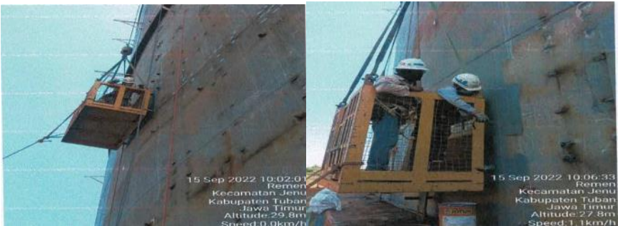
Fig. 5. Propane storage tank T-201 shell measurement using string line
