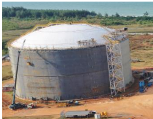
Fig. 1. Propane storage tank T-201 under construction
