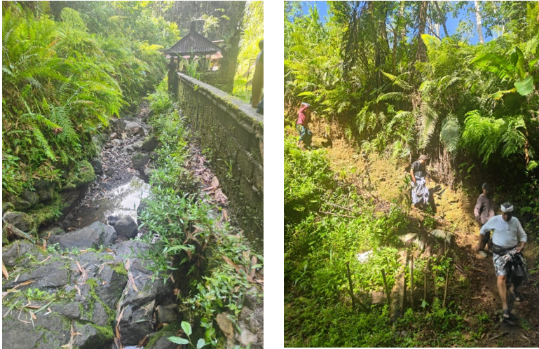
Figure 1. Existing Condition of Pura Luhur Pucak Les
