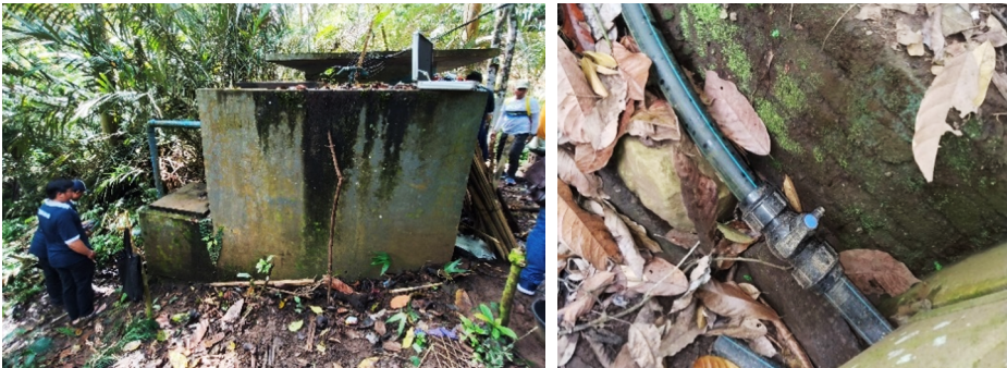
Figure 2. Existing water source, lower reservoir, pipeline route, and upper reservoir condition.
