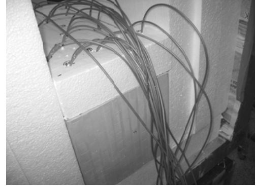
Fig.3: Thermal insulation of the brick block in the measuring system, sensors placing
