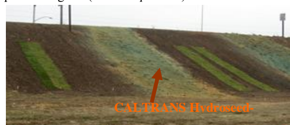
Figure 2 View of the Caltrans Hydroseed treatment on the highway fill-steep slope in November 2006.
