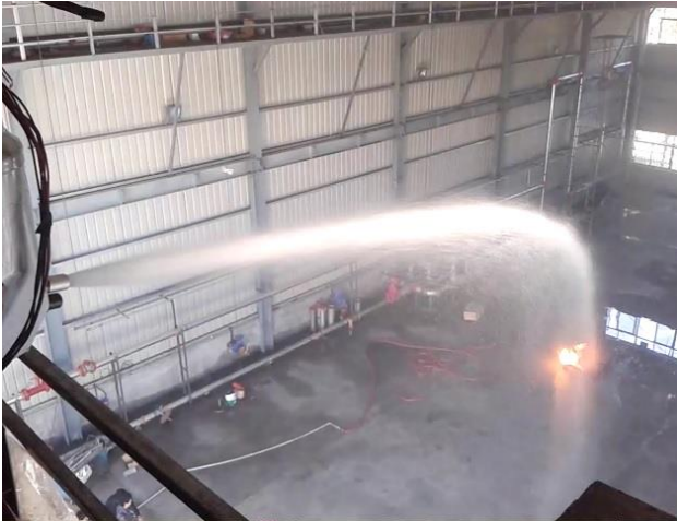
Figure 7. The test for automatic jet fire extinguishing device.
