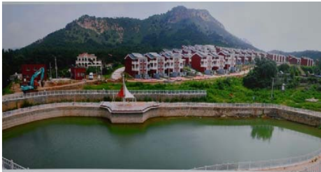
Figure 2. Pool of reclaimed water reuse.
