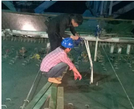
Fig.3 Temperature field testing
