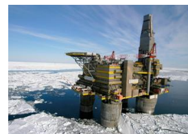
FIGURE II. OIL AND GAS PLATFORM IN THE ICE COVER.
