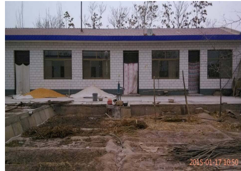
(b) New brick masonry residence
