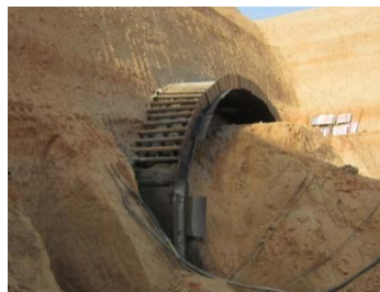
Fig.1 Construction of guiding umbrella arch in loess tunnel
