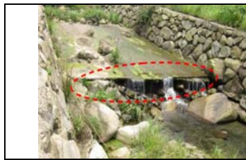
Figure 1-1. Groundsill work NO.1
