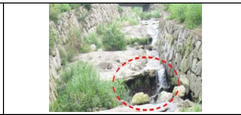
Figure 1-2. Groundsill work NO.2
