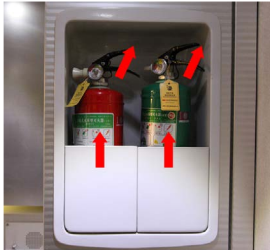
Fig. 1 The fire extinguishers and the box on high-speed train
