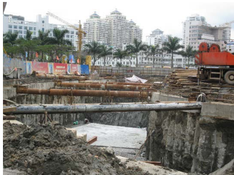
Fig.2 On-site photos of supporting structure
